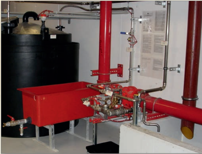
FD4000/1-PP-S in a sprinkler system with proportioning for protection of a high rack warehouse
