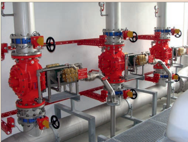
FD8000/3-PP-S in a deluge system with foam proportioning for protection of an aircraft hangar
