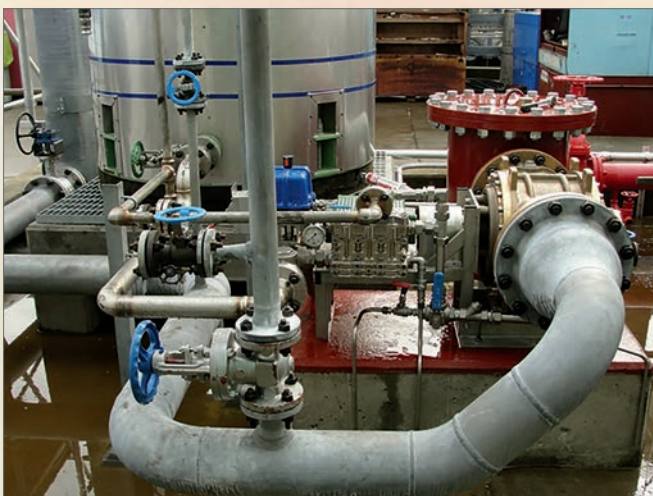
FD8000/1-PP-S seawater in a foam extinguishing system for protection of an oil loading terminal
