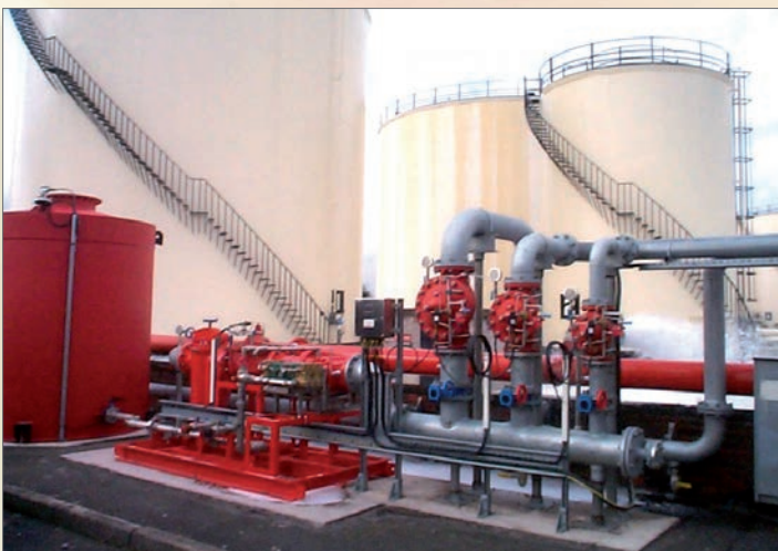
FD6000/3-PP-S in a foam extinguishing system for the protection of a tank farm
