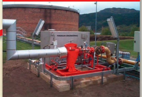
Foam extinguishing systems
