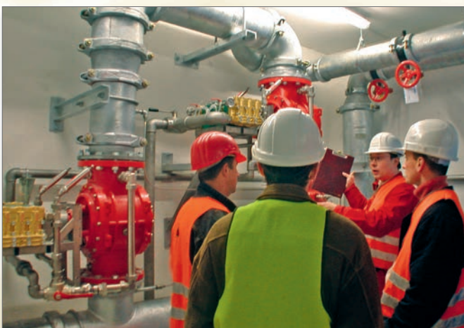
FD10000/3-PP-S and FD8000/3-PP-S in a sprinkler system with proportioning for protection of a painting line and painting preparation of an automotive manufacturer.
